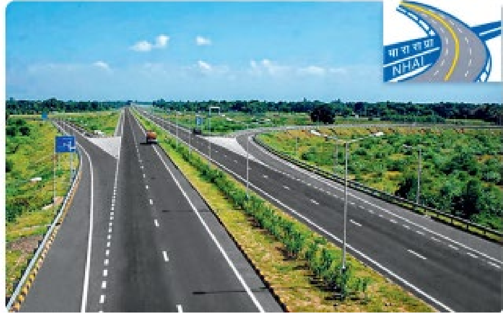
Land transport (Roadways)
