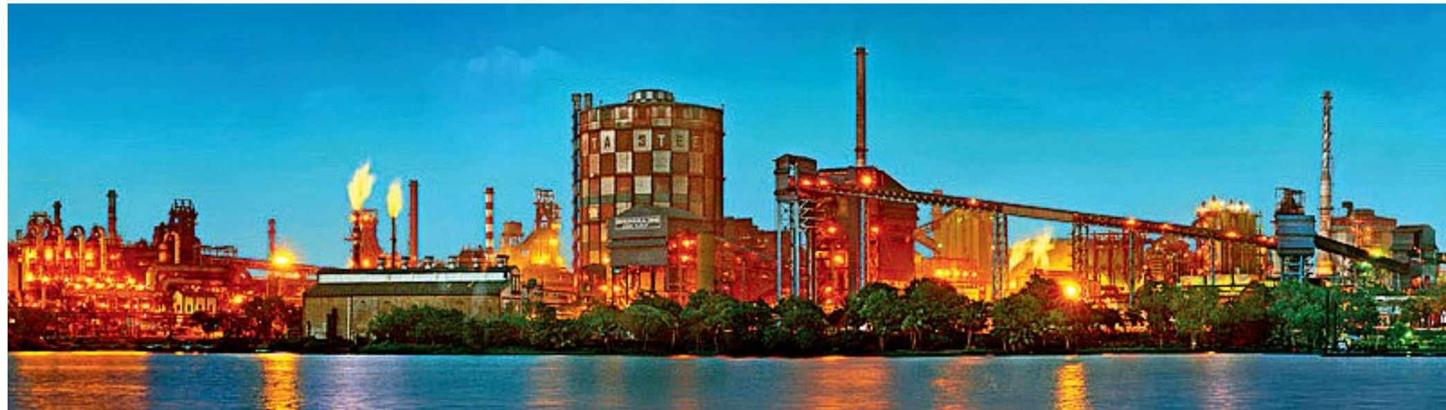
Iron and steel plant
