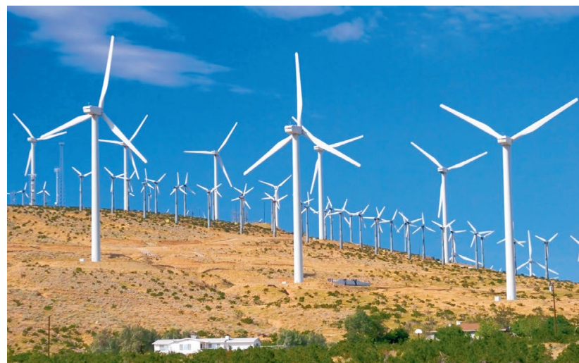
Wind energy farm
