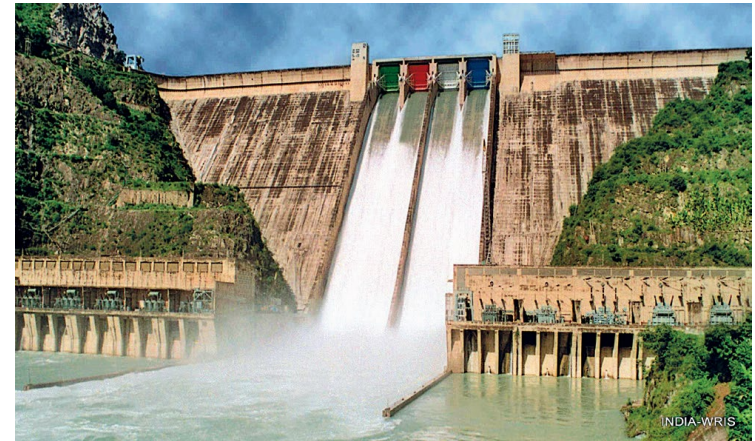
Bhakra dam on Satluj river
