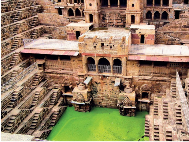
Baoli for water storage
