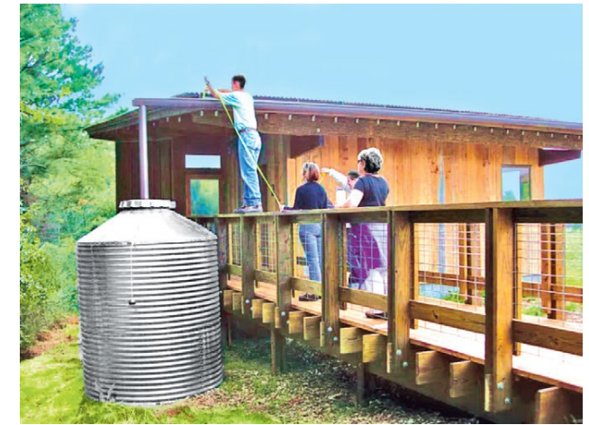
Rooftop rainwater harvesting
